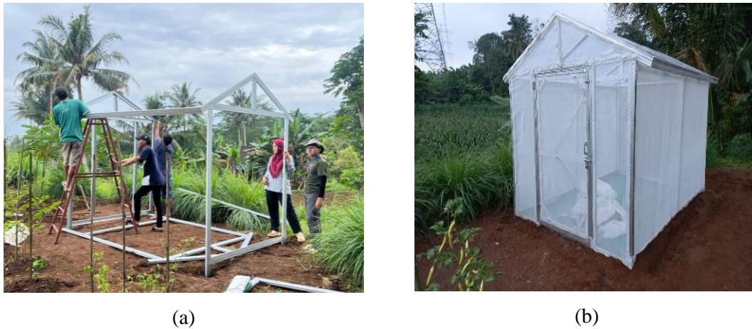
Fig 3. (a) Greenhouse Construction Process; (b) View of the greenhouse
